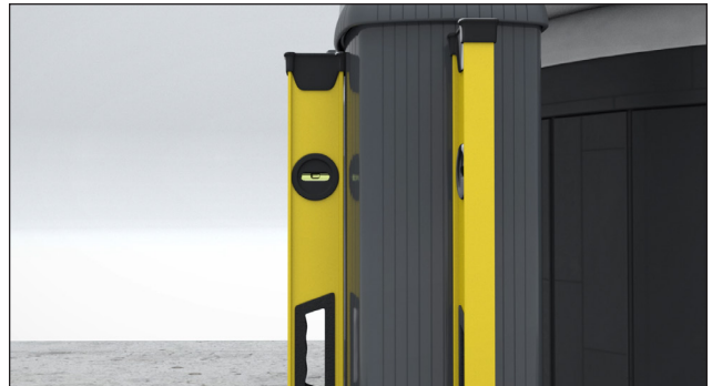
FIGURE 47: CHECK IF POSTS ARE STILL LEVEL
