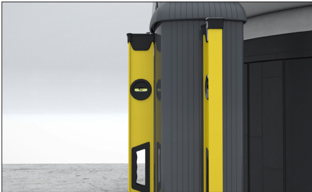
FIGURE 48: CHECK IF POSTS ARE STILL LEVEL
