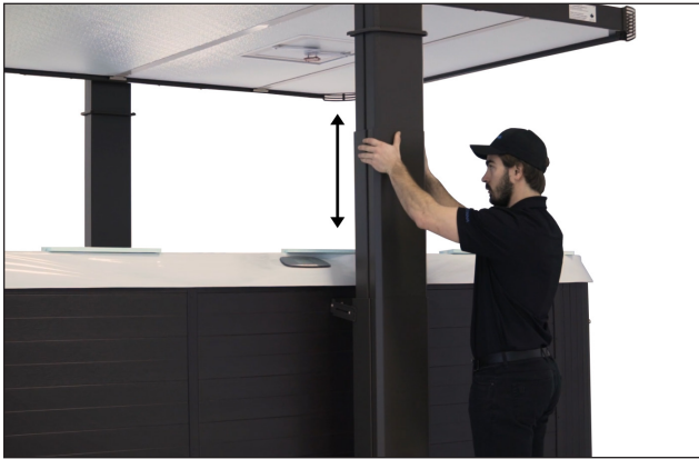
FIGURE 91: LOWER COVER AND CHECK IF THE SLEEVES ARE LEVEL USING A 36" LEVEL ON THE SIDE AND FRONT OF THE SLEEVES
