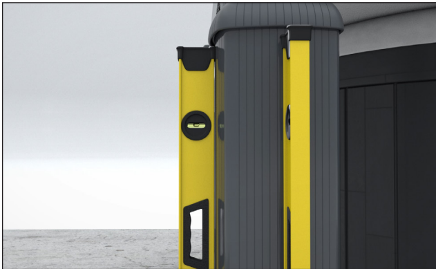
FIGURE 48: CHECK IF POSTS ARE STILL LEVEL
