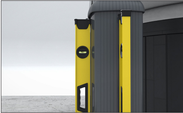
FIGURE 48: CHECK IF POSTS ARE STILL LEVEL
