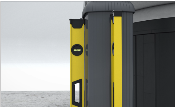
FIGURE 47: CHECK IF POSTS ARE STILL LEVEL
